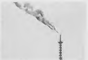
BRIGHT FLAMES indicative of flares are a common sight throughout the refining work. Flares are part of vast safety network that is effected during unit emergencies. VLAAMAN BRILLANTE cu indica presencia di flar ta un vista comun den benter mundo petrolero. Flares ta parti di un sistema grandi di seguridad.
